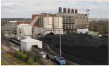
Figure 1. Potomac River Generating Station (2011)
